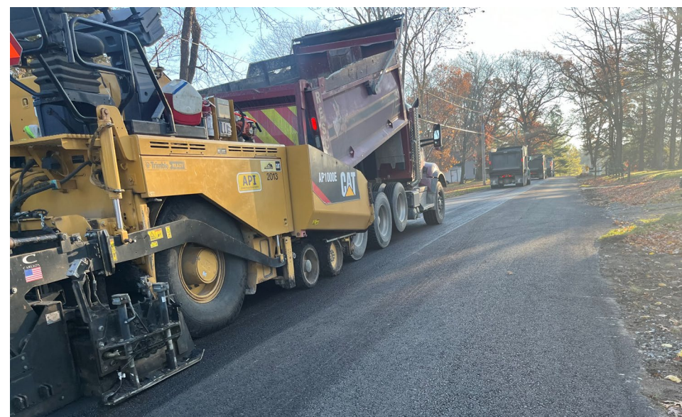
Looking East from 118 Lakeview, Paving 1.5" Surface Asphalt Layer
