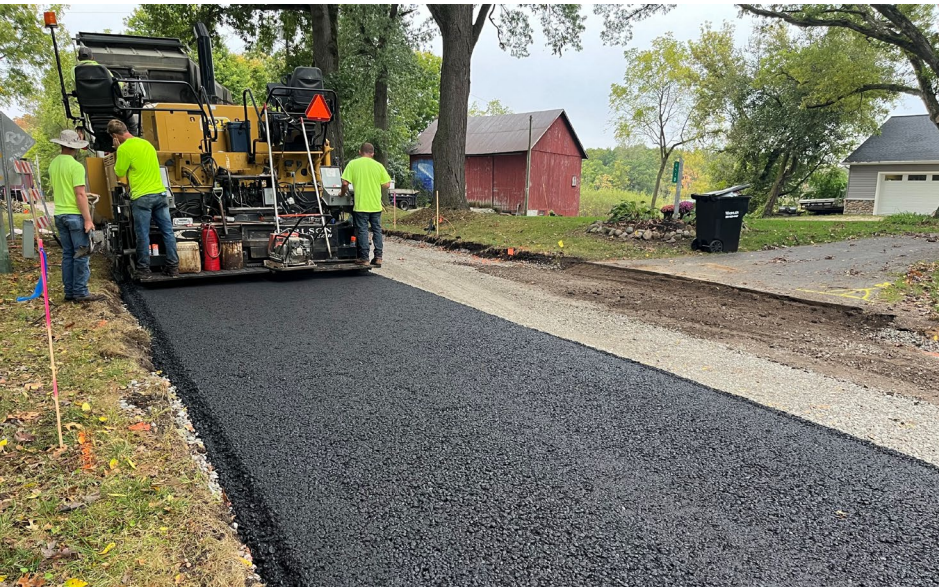
Looking West from 125 Lakeview, Paving 4" Intermediate Asphalt Layer
