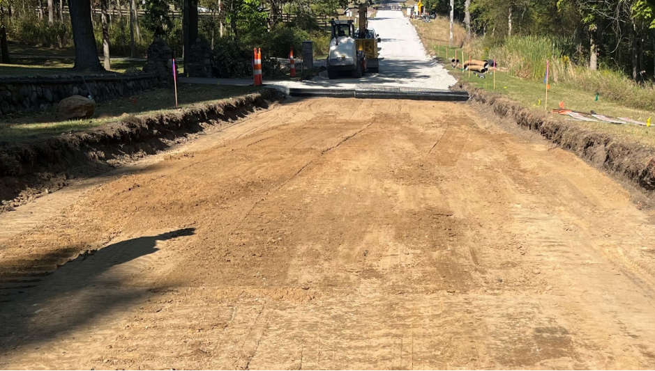
Looking West Toward Penner Dr from 114 Lakeview Showing Subgrade, and the Geogrid and Stone being placed heading East
