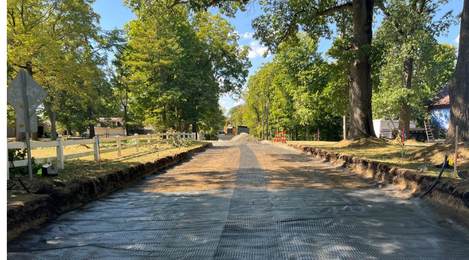
Looking West from 125 Lakeview, Geogrid is rolled out, some of this portion contains the Geofabric underneath, and Stone is being laid
